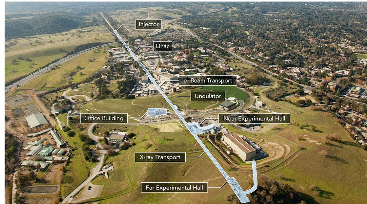
LCLS-II, Stanford, Aerial view
